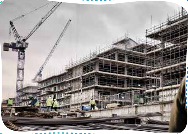
BUILDING SITE SECURITY
